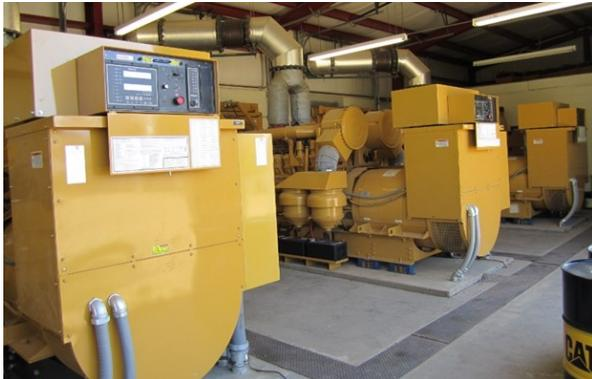
File photo - Caterpillar class engines, 1.2 MW capacity; Oxford
