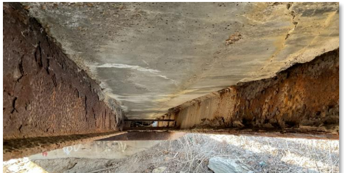
A look under the Palmer Road Bridge - 2024
